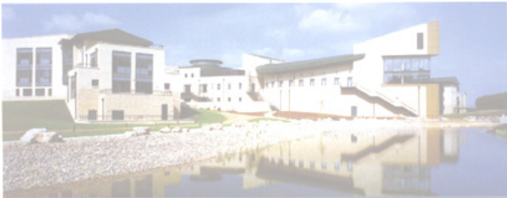
The wraps are off at HLM Architects' top-secret Joint Service Command and Staff College. The PFI scheme is valued at £500 million over 30 years and brings together the Army, Navy and Air Force in a giant 44,000m 2 combined residential training facility at Swivenham, near Oxford. The building is designed around a series of south-facing courtyards and features a library, mess and a 450-seat conference centre. HLM chairman Chris Liddle, is profiled on page 24.
